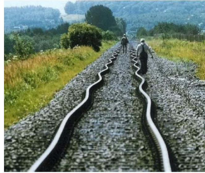
Track shift after a test run (O. Polach)
