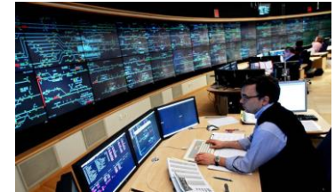
Traffic Control Centre
